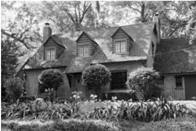
This vernacular home, located on Oakland Avenue, was built of brick and is classified as masonry vernacular.
