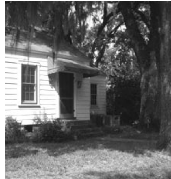
The awning above the front door on this Oakland Avenue home is fitted to the size of the door and does not overwhelm the front facade features. As a result, it is a complementary addition to the home.
